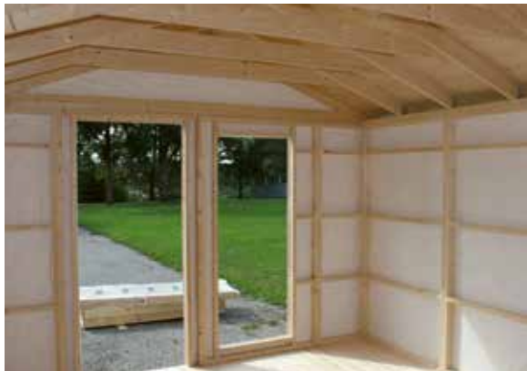
Internal view, walls covered with wind-protection film
